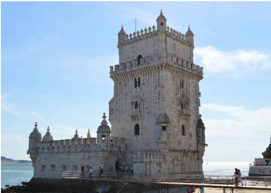
Turm in Betlehem
